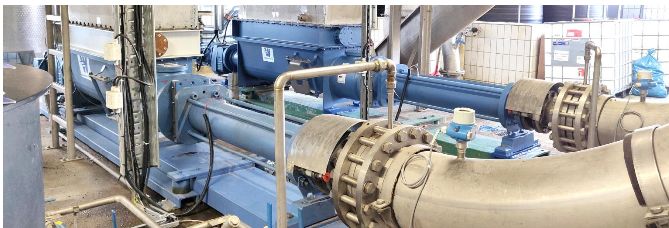
Installation of the pump in the system
