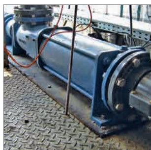
Pumping substrate between fermenters
