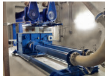
Conveyance of dewatered sewage sludge: KL80RQ110.4+110.4 Progres- sing cavity pump
