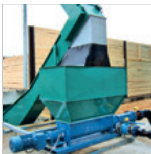
Feeding the pump via a transferring hopper
